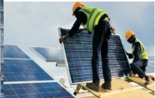
Solar Power Installation
